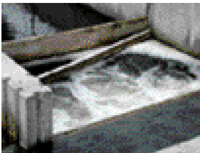
Double screen system on the inflow is useful where surface water sources may carry substantial amounts of debris
