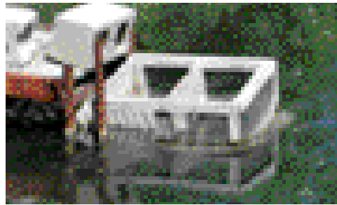
A box type screen installed on rearing pond outflow increases the surface area of the outflow pipe
