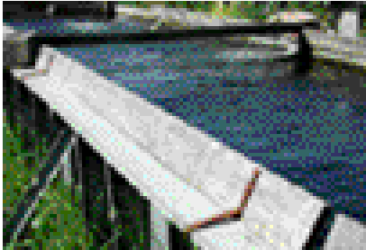
Simple attachment of angled boards to block jumping
